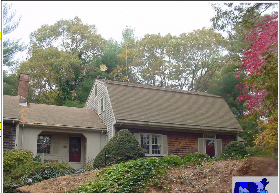
72 S STATION ST
