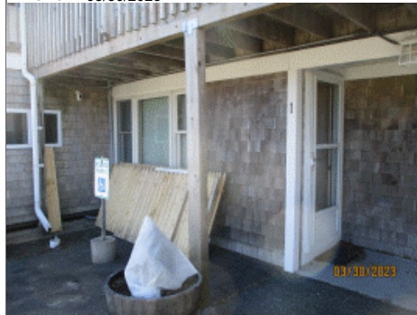
UNIT 1 = GROUND LEVEL TO RIGHT OF OFFICE & MGR'S QUARTERS
